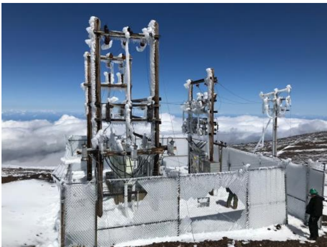
The summit's power substation was draped in ice and surrounded by snow during severe conditions. MECO photo
