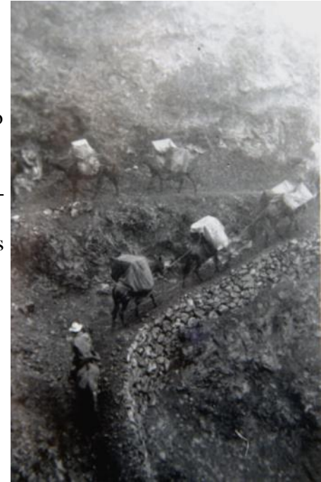
Mules haul supplies for early park construction projects.
